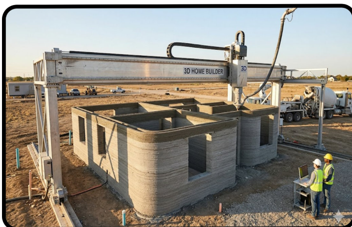
A house being 3D printed
